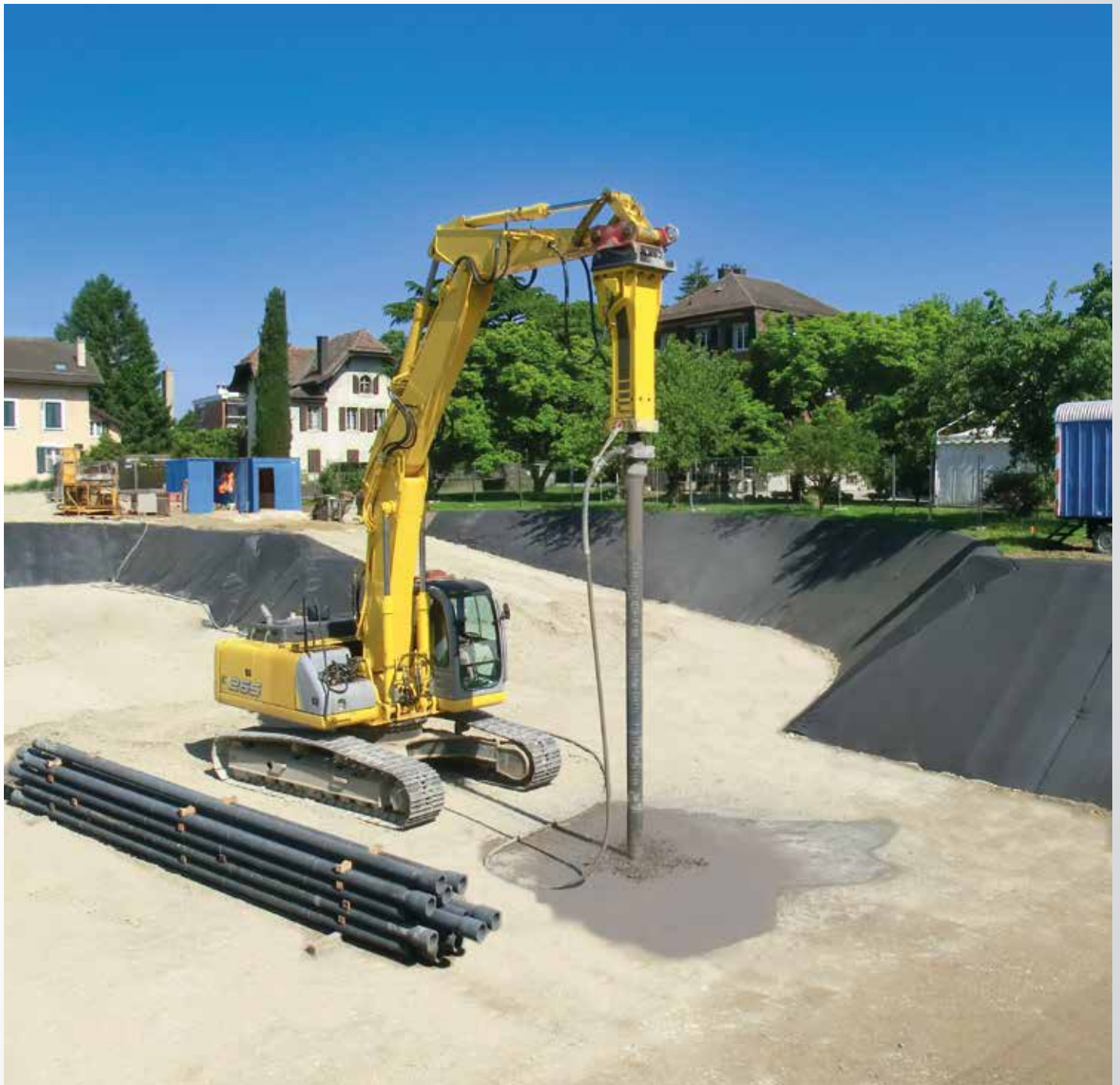
A stable foundation.
