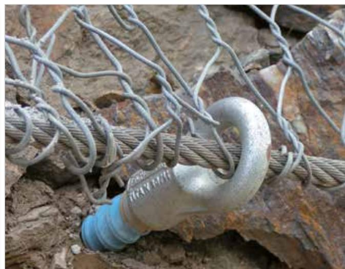
Pile head detail with hot-dip galvanised **eye fitting** for holding wire ropes
