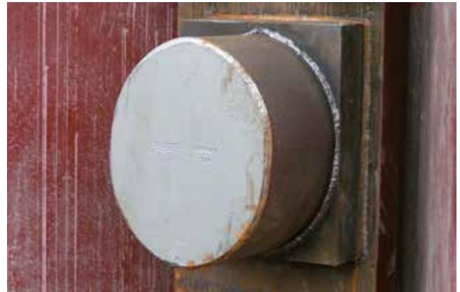
Pile head detail with protection cap
