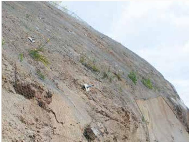
After installing the hollow bars, the surface was secured with wire mesh held in place on the slope with spherical collar nuts and domed claw washer plates.
