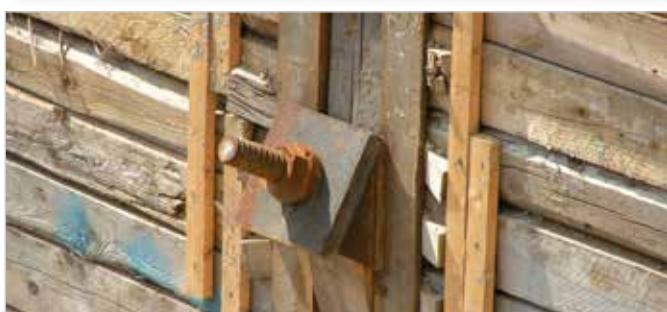
Excavation shoring anchored with TITAN 40/16 and TITAN 52/26 without walings
