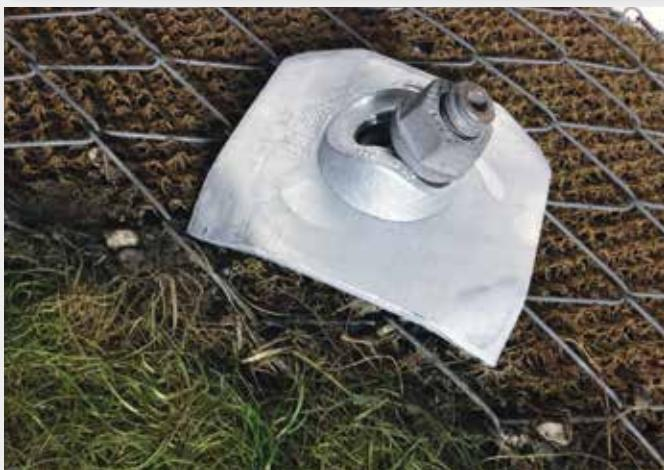
Differences in angle of up to  $+36^\circ$  between nail and terrain can be compensated for by fitting a self-centring TITAN angle adaptor plate (shown here with domed claw plate).
