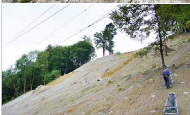
An unstable embankment more than 20 m high stabilised with soil nailing and secured with high-strength wire mesh.
