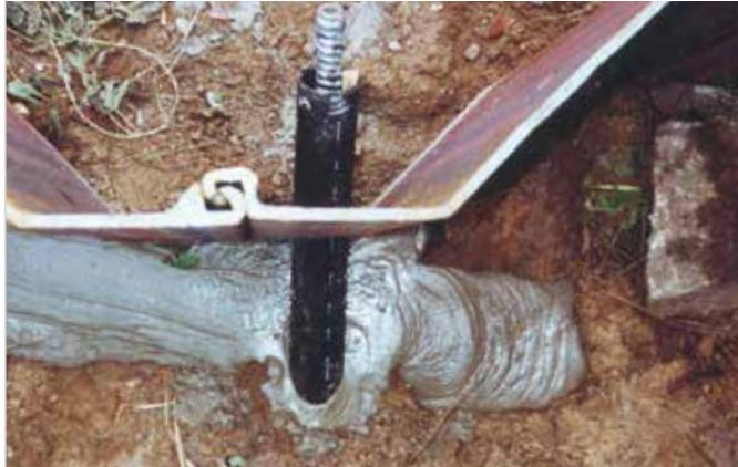
An HD-PE or steel tube to suit the structural requirements protects the hollow bar against damage and corrosion when backfilling behind the sheet pile wall.
