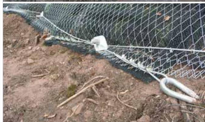
**Flexhead** for fixing wire ropes
